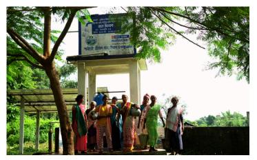
Jal Minar is a marvel of engineering, combining a 10,000-liter storage tank with a solar-powered pumping system- a 3 HP solar pump, fueled by a powerful 3,000-watt solar panel.
